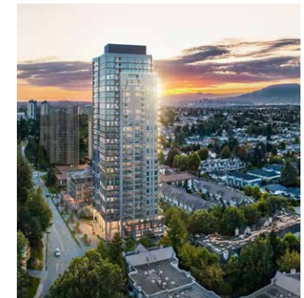
ARTESIA METROTOWN By Qualex-Landmark 247-unit 31-storey high-rise
