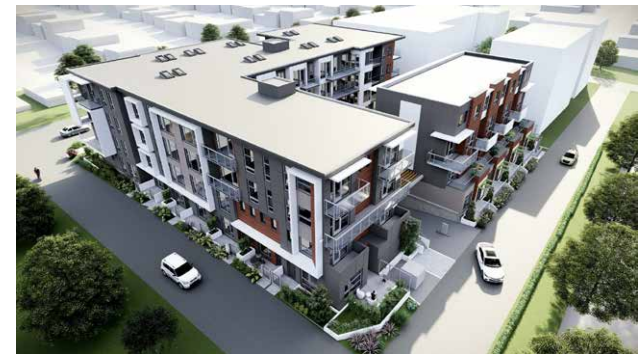
SOUTH WEST LANE VIEW
