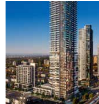
HIGHLINE By Third Properties 327-unit 48-storey high-rise
