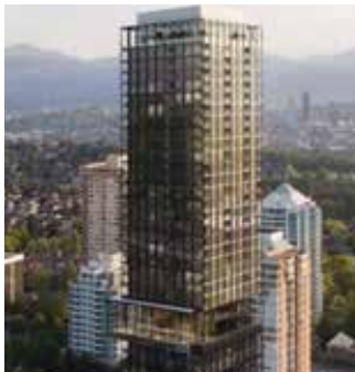
CENTRAL PARK By Bosa Properties 335-unit 39-storey high-rise
